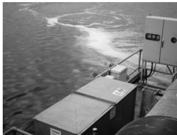
Figure 7: Oxygen injection into Salford Quays.
